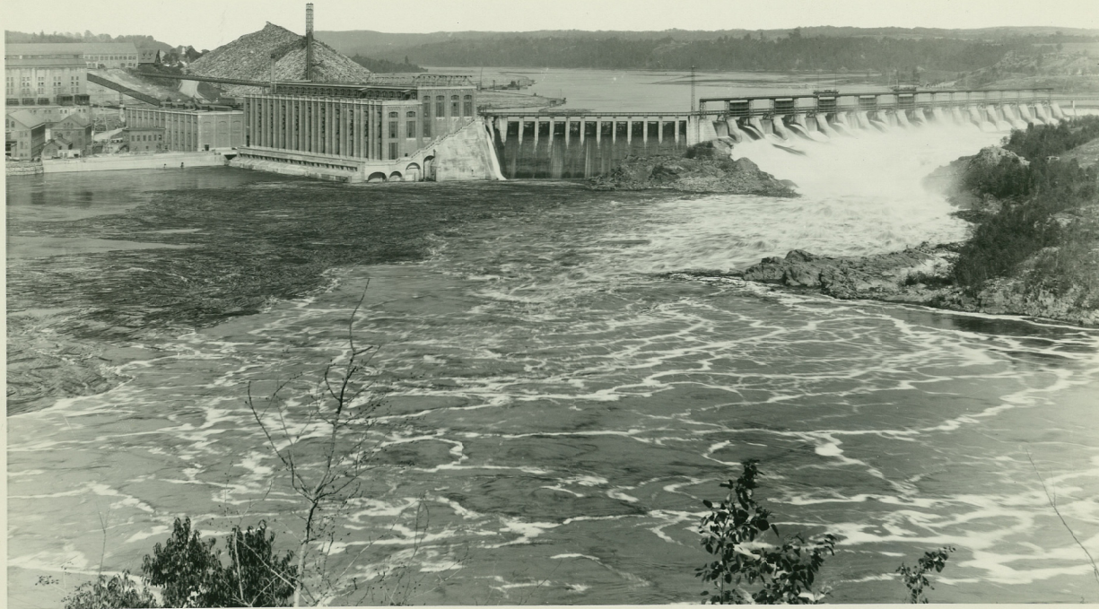
GRAND'MERE PLANT View of Power House and Dam from Tailrace
